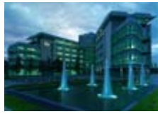
The new corporate head-quarters, the Adam Opel Building in Rüsselsheim, 1998.
